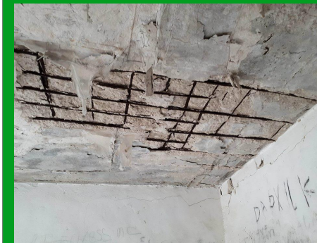
All exposed reinforcement bars must be thoroughly cleaned and apply suitable protective prime. Apply slurry(bonding coat) to all concrete surfaces to which bond is required
