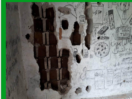
Hack and remove all eroded plaster. Provide cement plaster for all walls and paint to approval
