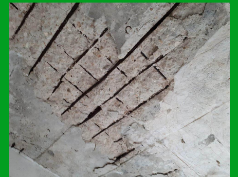
All exposed reinforcement bars must be thoroughly cleaned and apply suitable protective prime. Apply slurry(bonding coat) to all concrete surfaces to which bond is required
