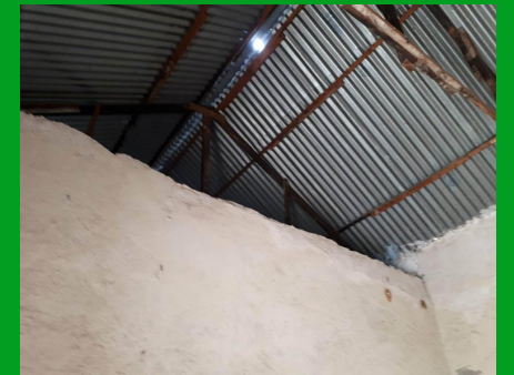
All asbestos roofing shall be removed (together with timber frames) and replaced with GI
