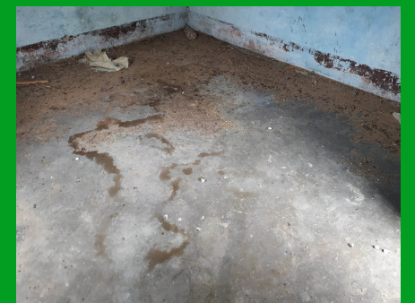
All cement screed floor shall be repaired according to specifications
