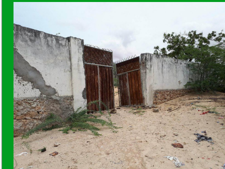
View of boundary wall. The wall is damaged in some segments.
